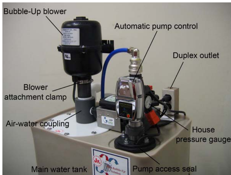
Fig. 2A Installation Points
